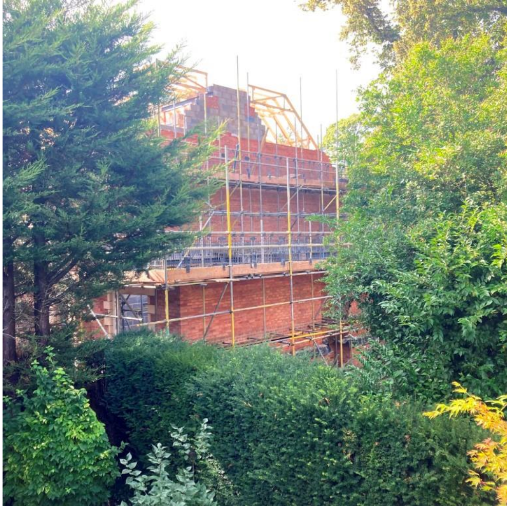
Vertical gable under construction, 24 August 2024
